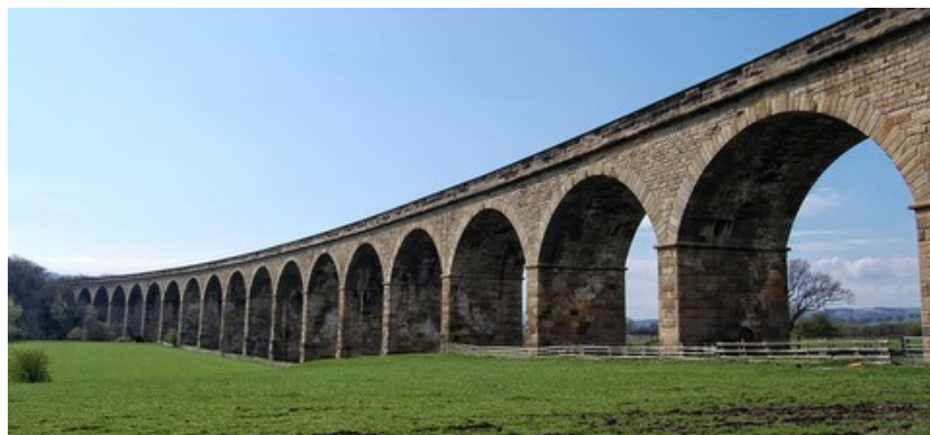
A viaduct consisting of a continuous regimented row of vertical columns and arches.
