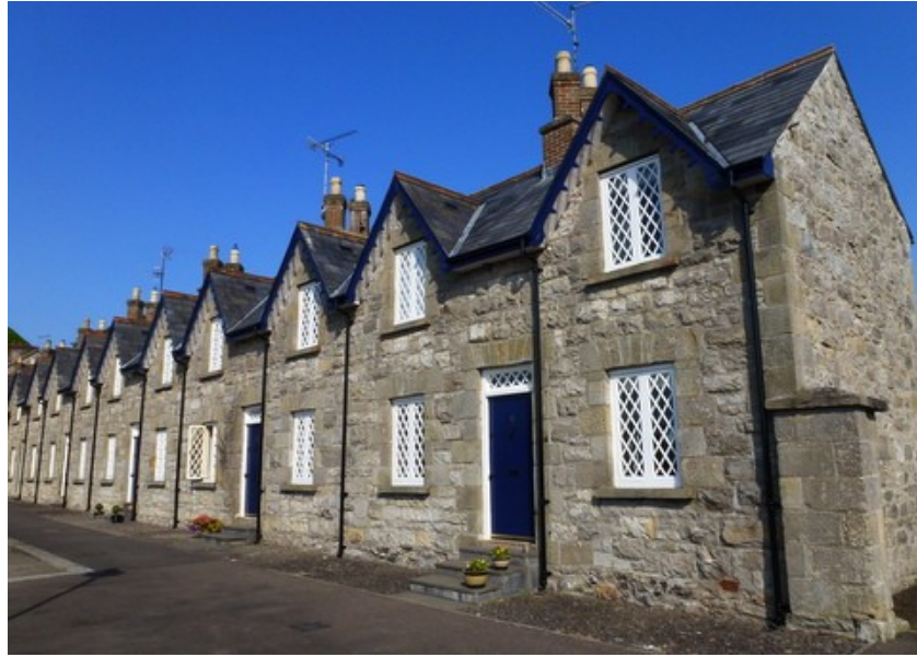
A row of cottages with a continuous row of regimented vertical doors and windows with each one sitting within its own bay. Stone quoins on the corners, stone surrounds around each aperture and a complete row of chimney stacks and all doors the same colour.
