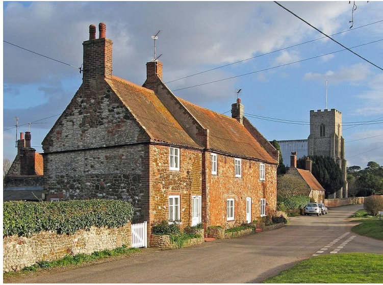
Hunstanton: Red-brick, with lime, sand and cobblestone mixed, roofed with pantiles with higher gable-ends.
